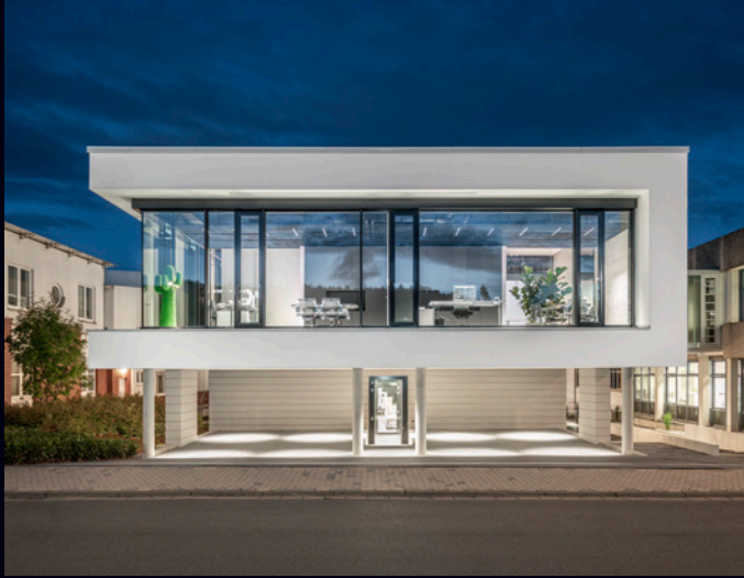
Headquarters in Arnsberg
